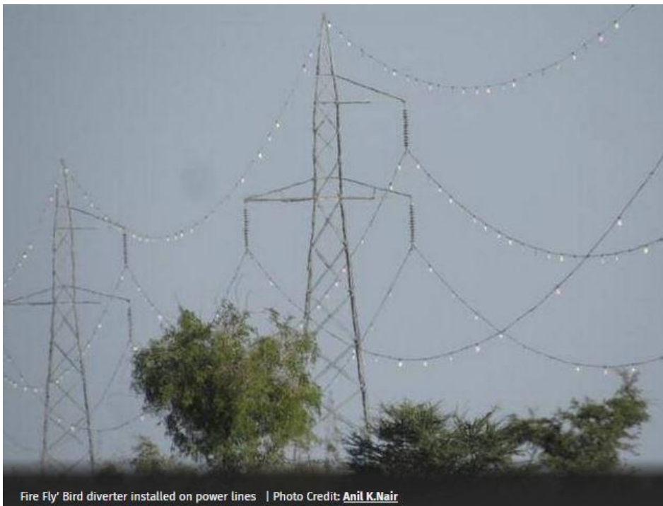
Fire Fly Bird diverter installed on power lines | Photo Credit: Anil K.Nair
